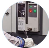
Levering Magnum DS breaker through the door
