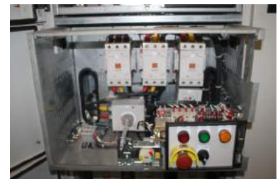
Front view of a withdrawable motor starter unit up to 37—55 kW (380 mm).
