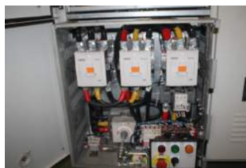
Front view of a withdrawable motor starter unit up to 75—110 kW (580 mm).
