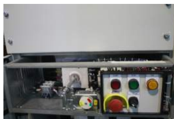
Front view of a withdrawable motor starter unit up to 15—30 kW (180 mm).
