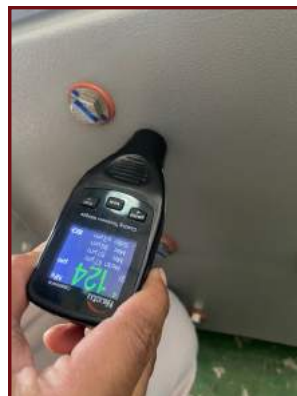
Paint Thickness Check
